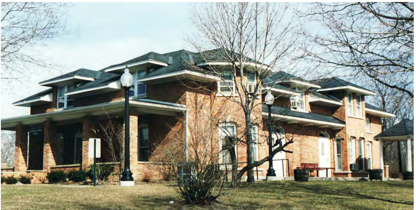
The structure has served the City of Dearborn as a Museum for over 60 years.
