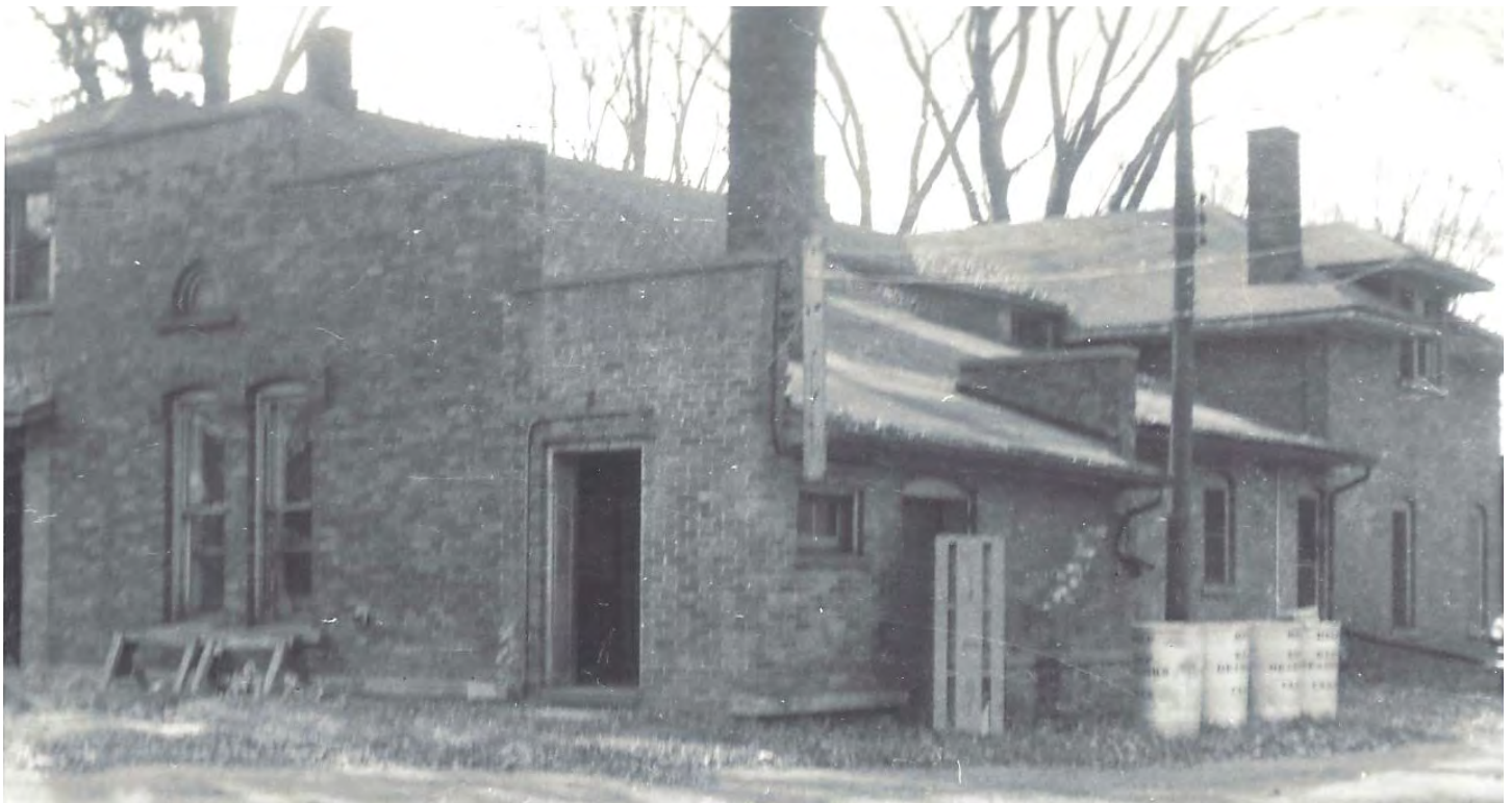
A view of the back exterior before alteration. The kitchen area just inside the doorway was torn down, a back stairway installed and the roof extended with a dormer put in to create another meeting room upstairs.
