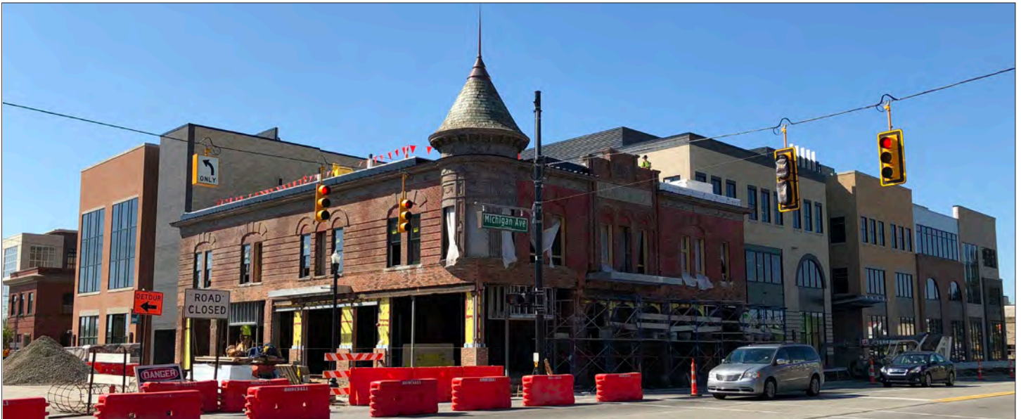
The Wagner perseveres even while surrounded by 21st Century office buildings. Photo/Millard Berry
