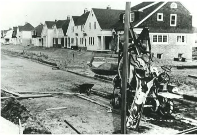
Ford Homes used production line methods originally developed for the automotive industry.
