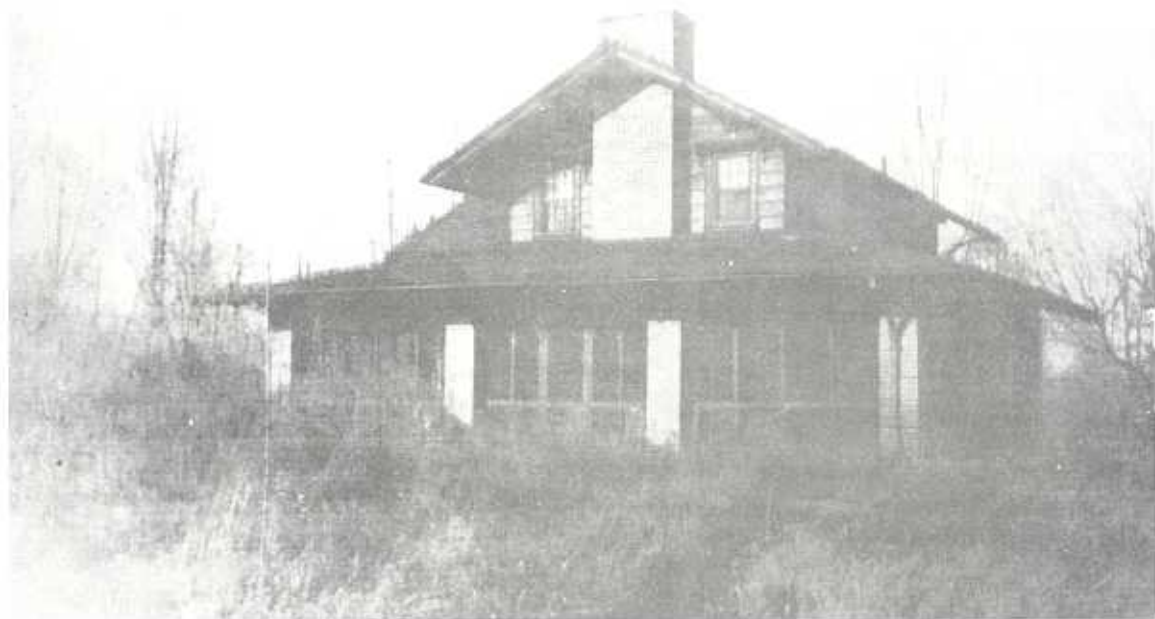
November, 1912, picture of the "Bungalow" built in 1909 by the Fords as a weekend retreat from the city. It was located on the west bank of the Rouge River about a third of a mile upstream from the Black farmhouse. It was close to the present site of the First Presbyterian Church on Brady Street, north of Cherry Hill. (Photo from the Edward L. Bryant collection.)
