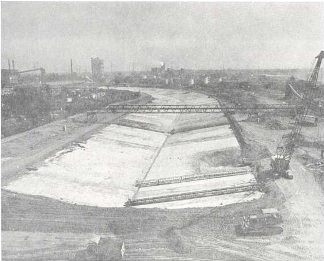
Paving of the River Rouge in the area of the Ford Motor Company's Rouge Complex. Courtesy: Dearborn Times-Herald .
