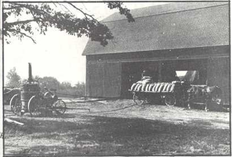
Above: Soy bean threshing time at a Ford Farms barn - 1930's. Machine at left is a steam thresher.
