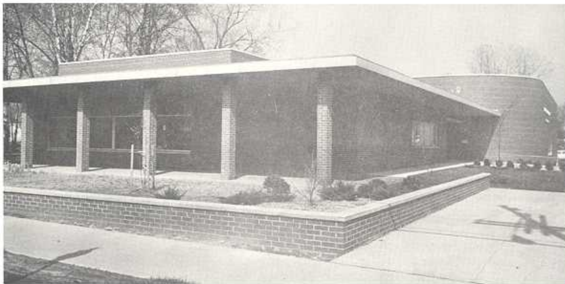
Exterior of the Clara L. Snow Branch, 1965, located at 23920 Princeton.
