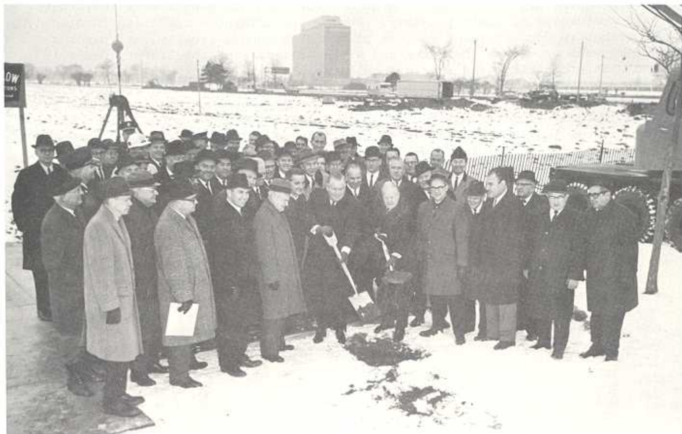
Ground-breaking ceremonies for the Henry Ford Centennial Library, December 14, 1966. Present are City and Ford Motor Company officials. In the background is the Ford Central Office building, a Dearborn landmark.
